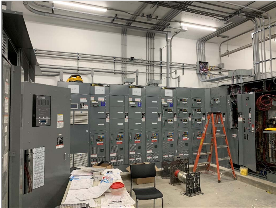
Electrical wiring mostly cleaned up, some control cabinets still underway.
