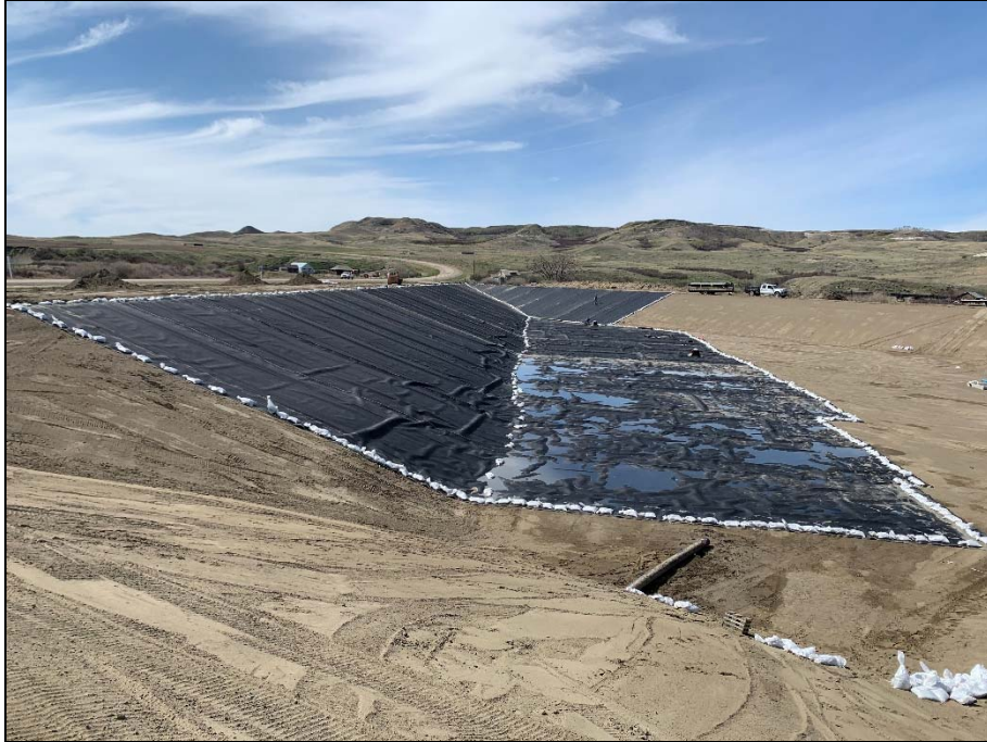
Reservoir liner installation.
