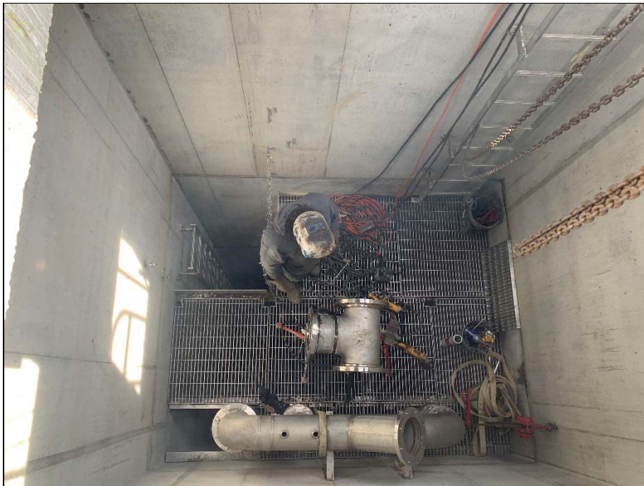
Welding work in river pumphouse.
