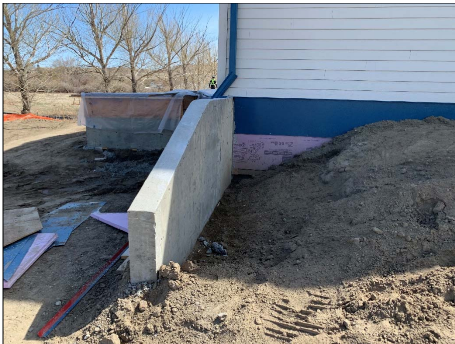
Retaining wall in place.
