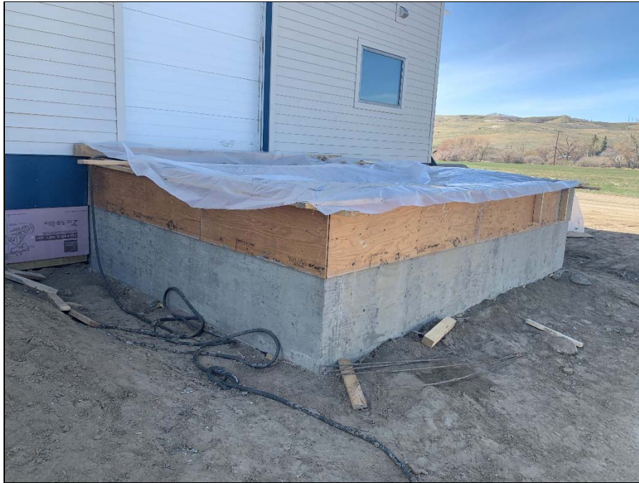
Loading dock grade beams completed; formed for top slab.
