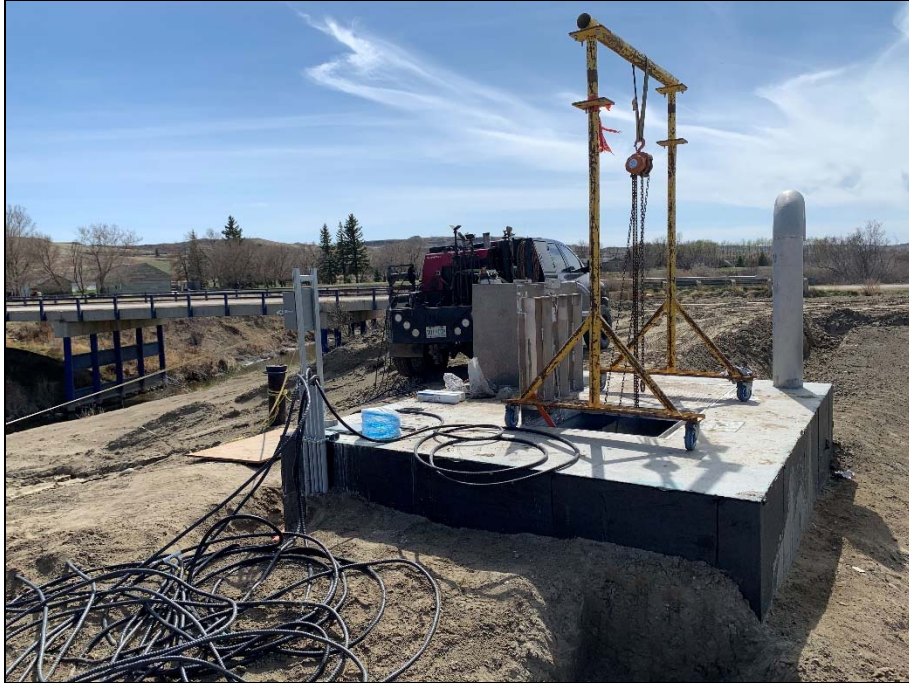
Mechanical and electrical work at river pumphouse.
