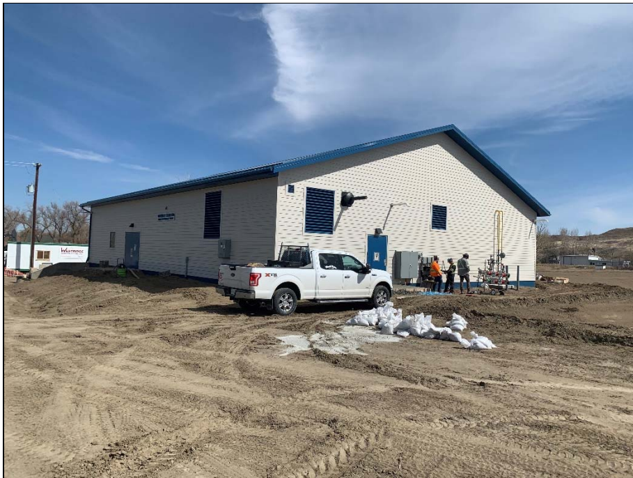
Electrical work outside building.
