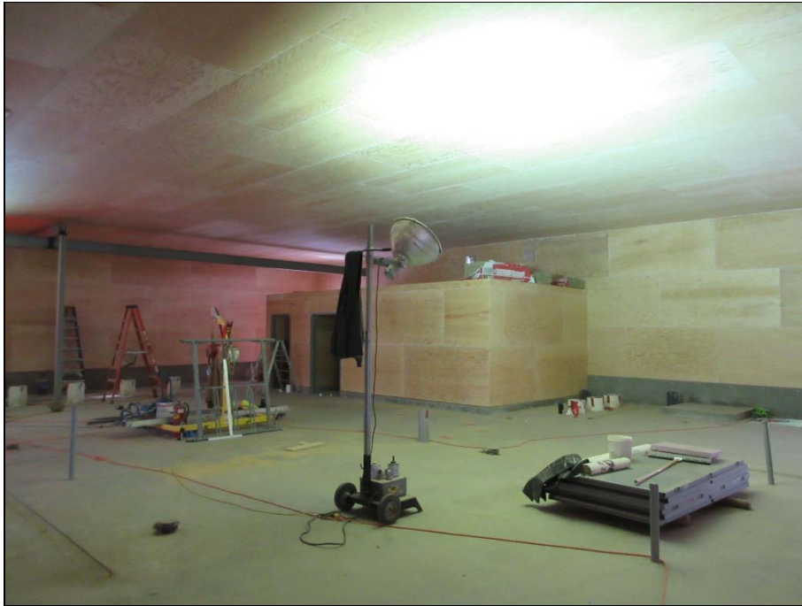
Building interior is framed and sheathed.
