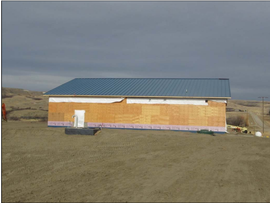
Rear of water treatment plant; insulation, flashing and roofing completed.
