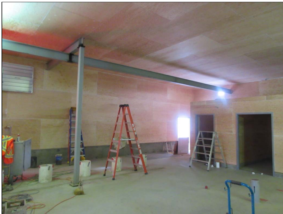
Overhead pump lifting beam in place.
