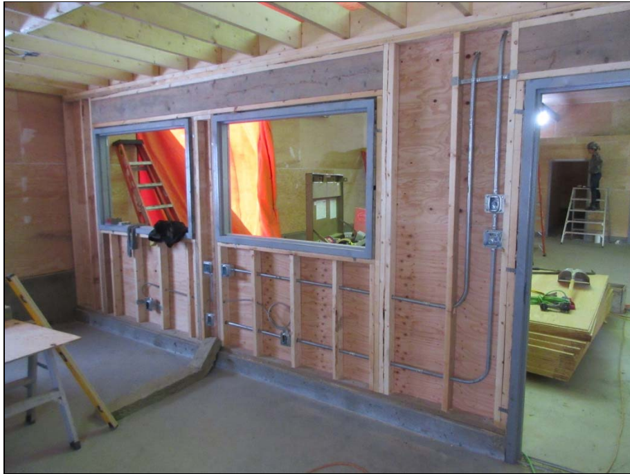
Office electrical rough in.
