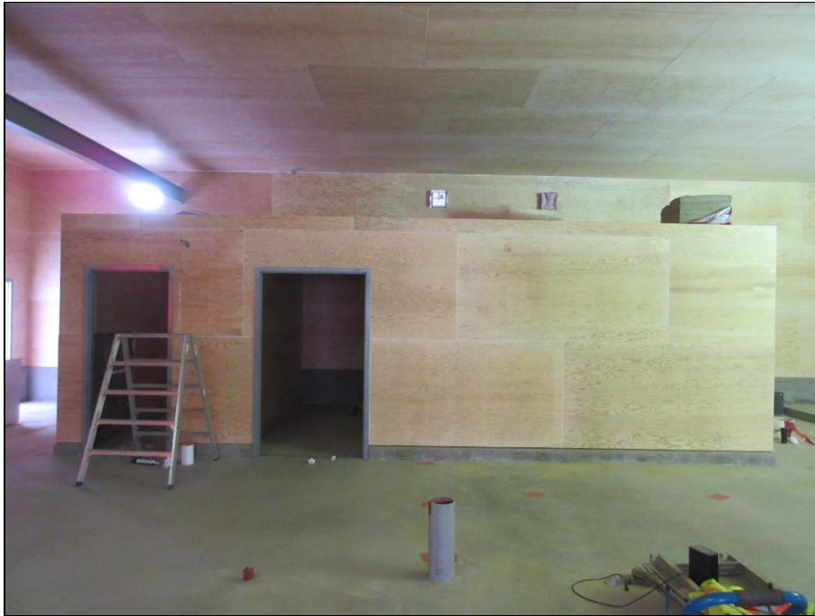
Washroom and chemical room.
