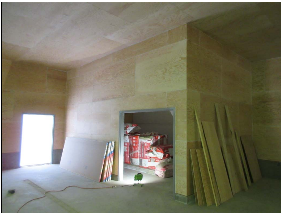
Generator room is framed and sheathed.
