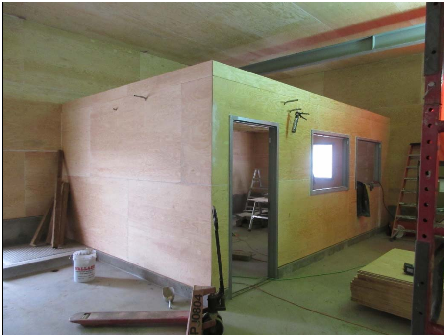
Office framing including door and windows.
