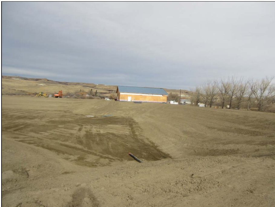
Earthen raw water reservoir excavation is completed.
