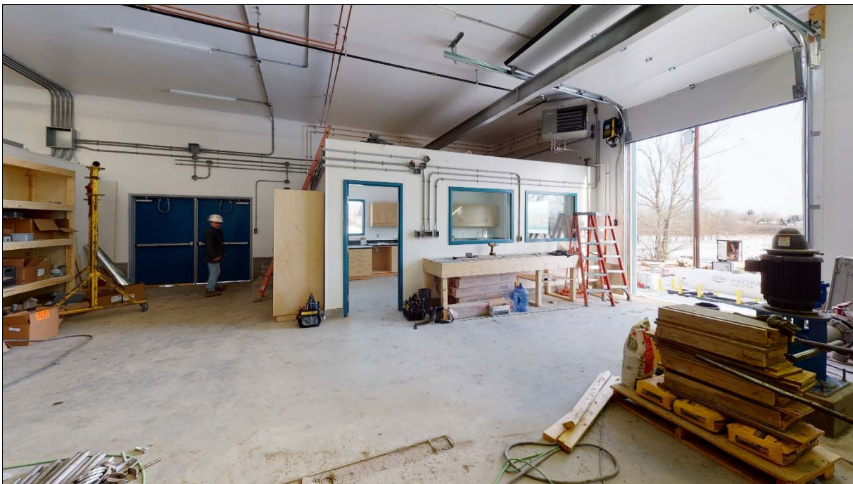
Office, overhead door, and work bench.
