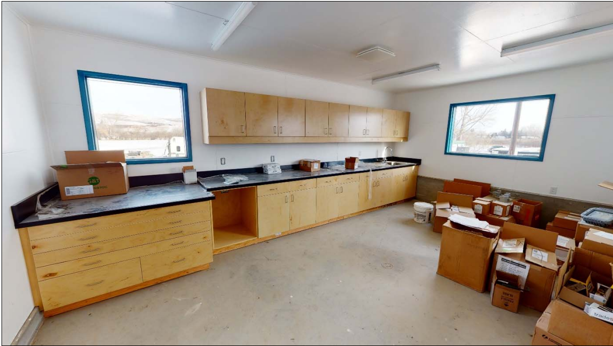
Office millwork is complete; office requires tiling and furniture.
