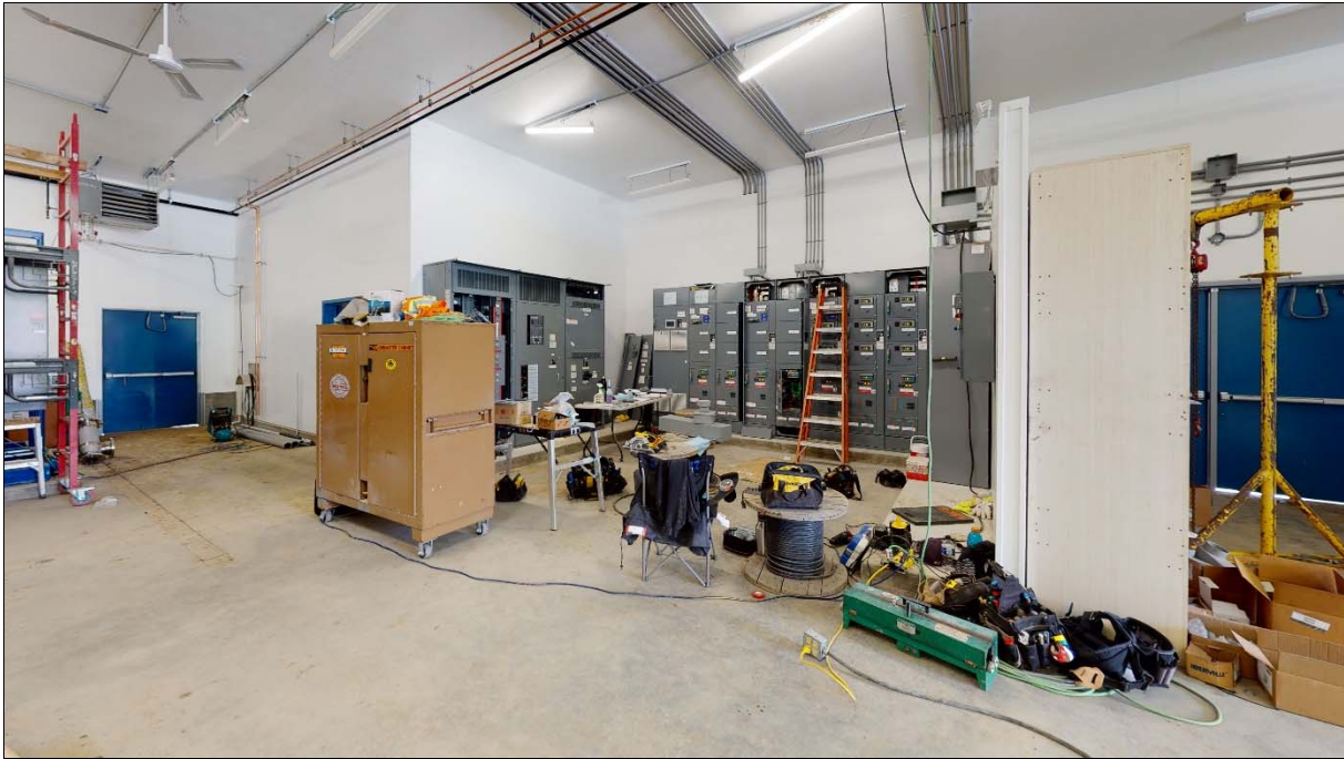
Electrical rough in and MCC work underway.
