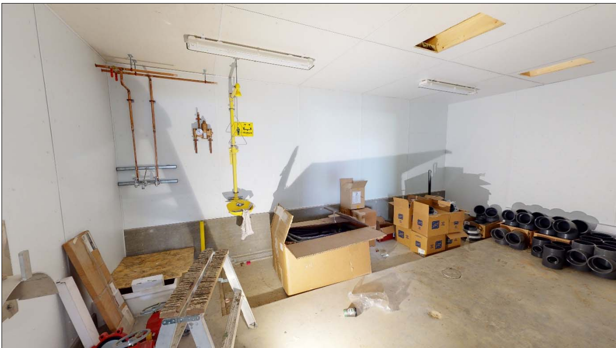
Chemical room construction / plumbing; cut-outs for ventilation fans in ceiling.
