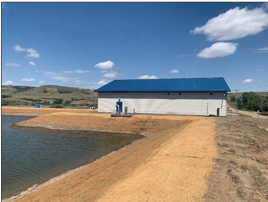
Erosion protection and seeding on interior face of raw water reservoir.
