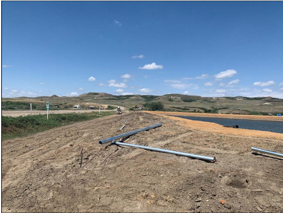
Chain link fencing starting; materials on site.
