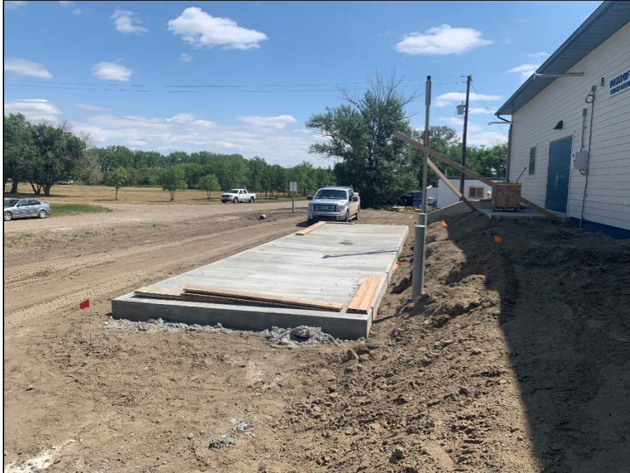
Truck fill slab and bollards in place.
