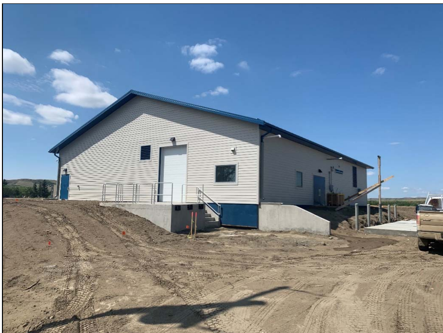
Nearing final grading around WTP to start roadway construction.
