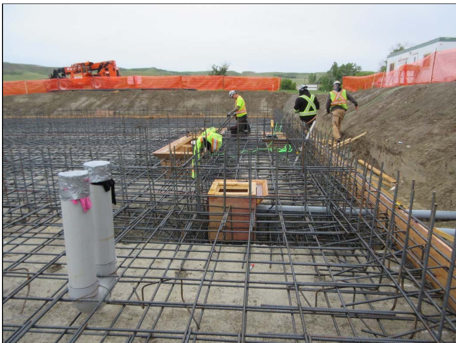
Bottom slab rebar inspection – sump boxes, wall dowels and pipe penetrations.
