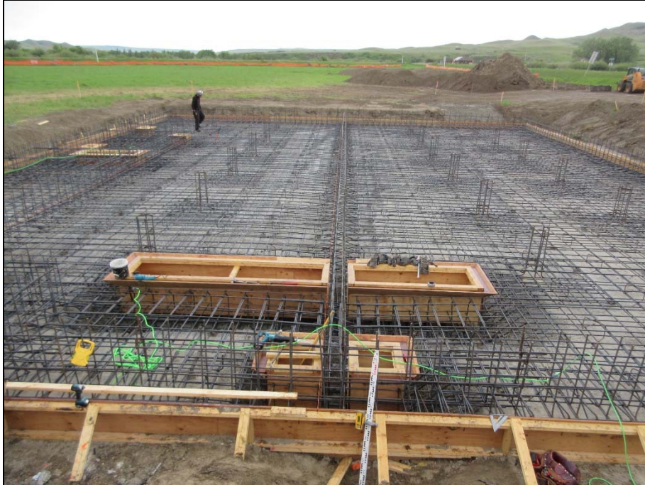
Bottom slab rebar inspection – overall view.
