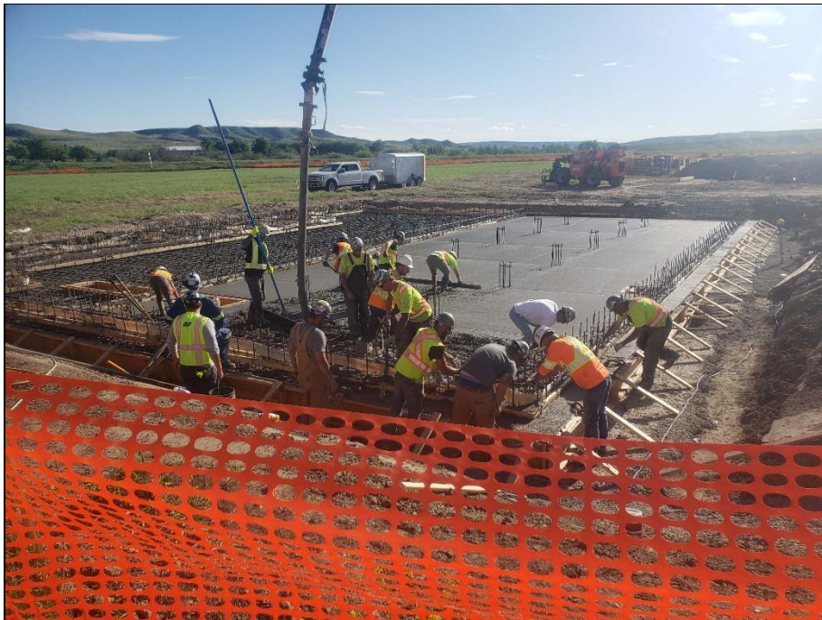
Bottom slab concrete pour underway – vibration and finishing work.
