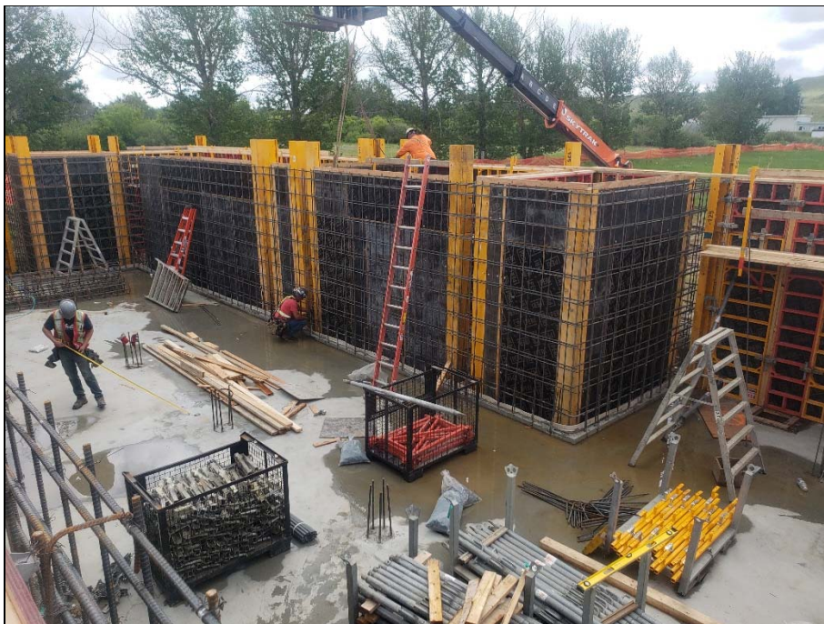
Wall rebar and formwork inspection – interior walls.
