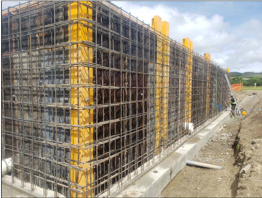
Wall rebar and formwork inspection – exterior walls.
