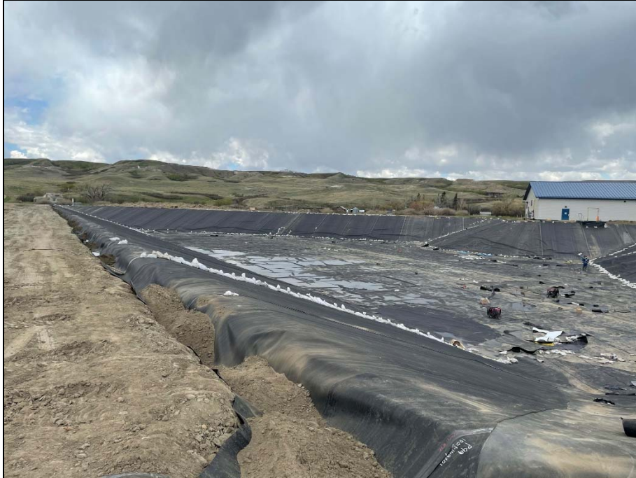
Liner installation completed.
