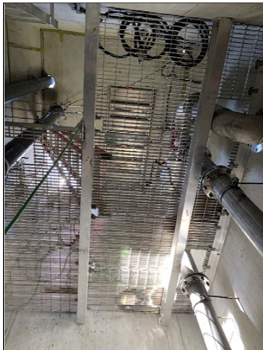
Intake pumphouse working platform (from below).
