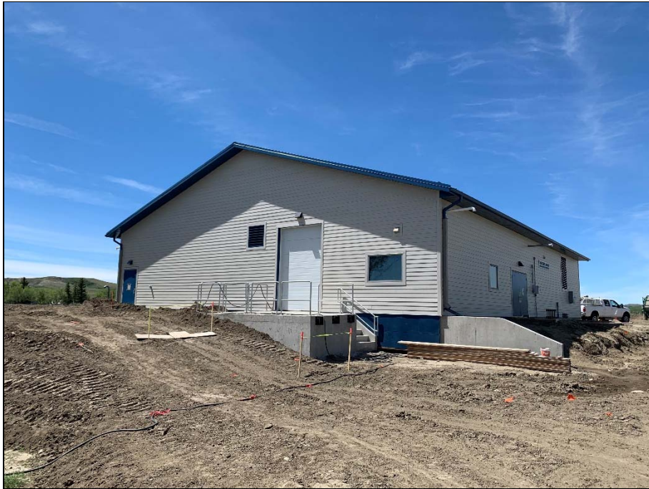
WTP exterior with loading dock completed.
