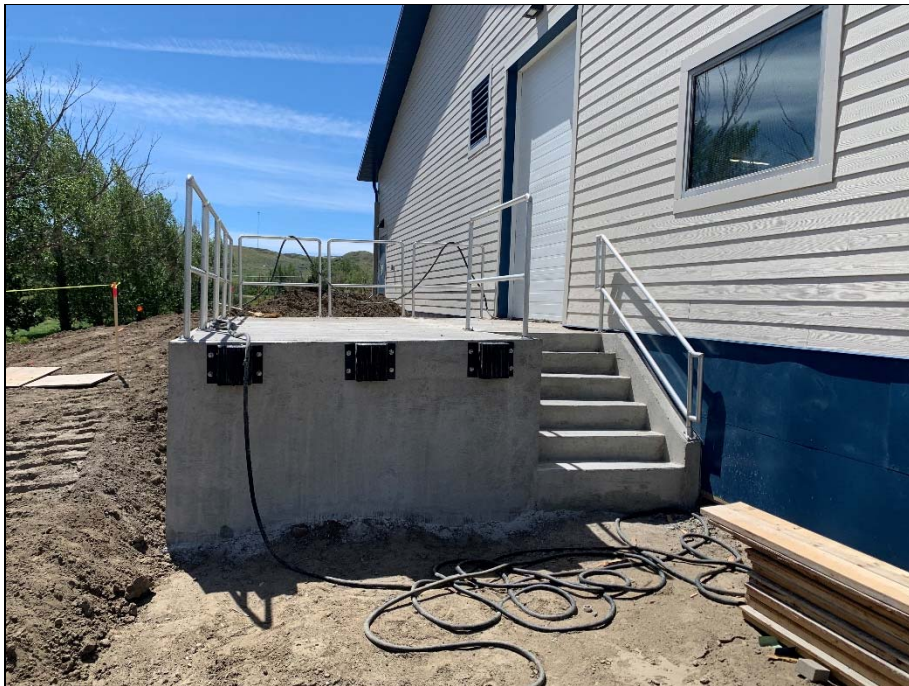
Loading dock, stairs and railings.
