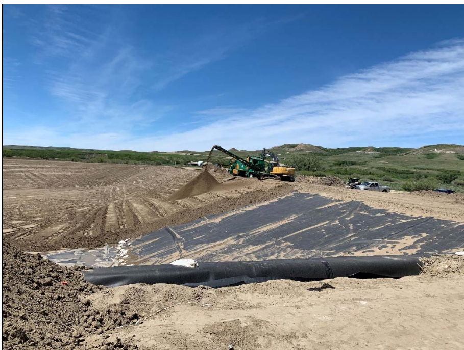
Liner cover installation ongoing.
