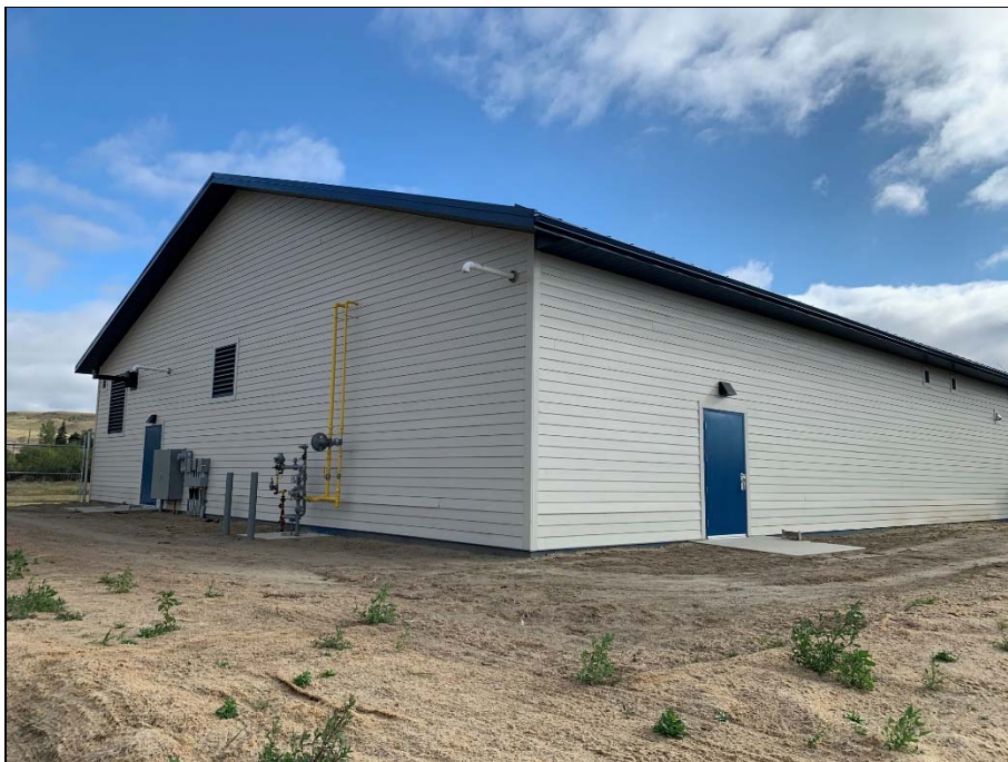
Rear of WTP.
