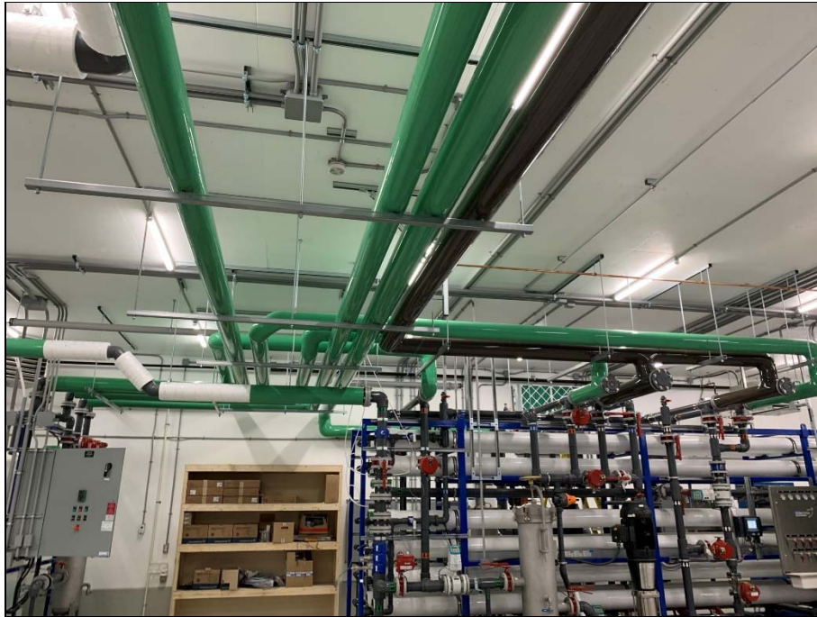
Piping insulation and colour coded jacketing work underway.
