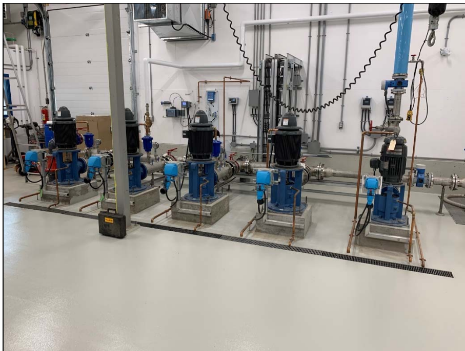
Distribution piping completed; floor epoxy coating applied.
