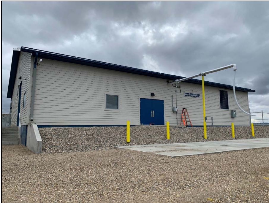
Front of WTP – truck fill station completed and bollard painting underway.
