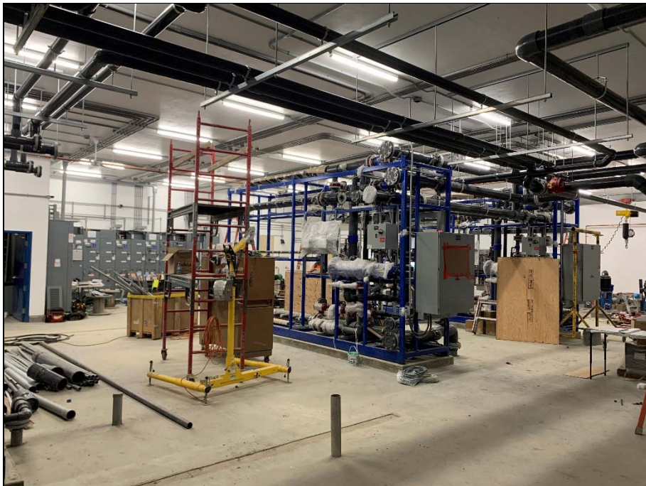
Most piping secured in place.
