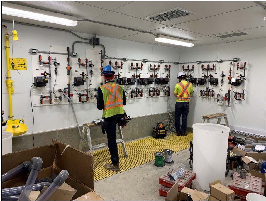
Chemical room equipment mounting underway.
