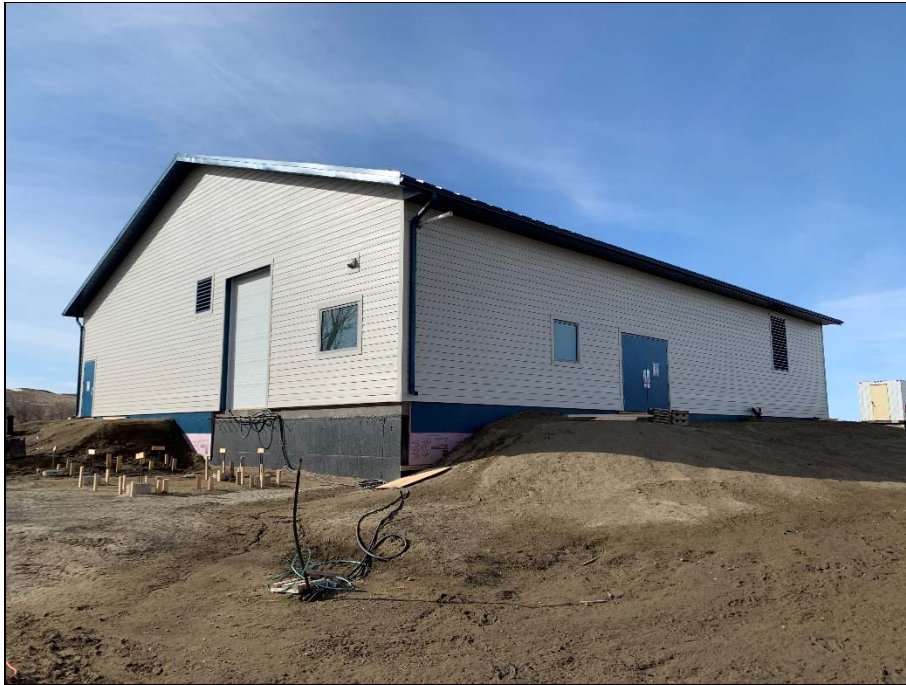
Plant exterior is completed except for loading dock on east side.
