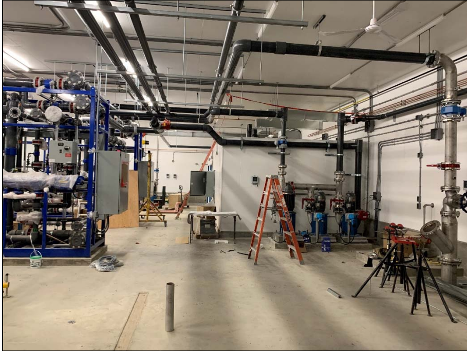
Significant progress on the pumps, piping and valves within the plant.
