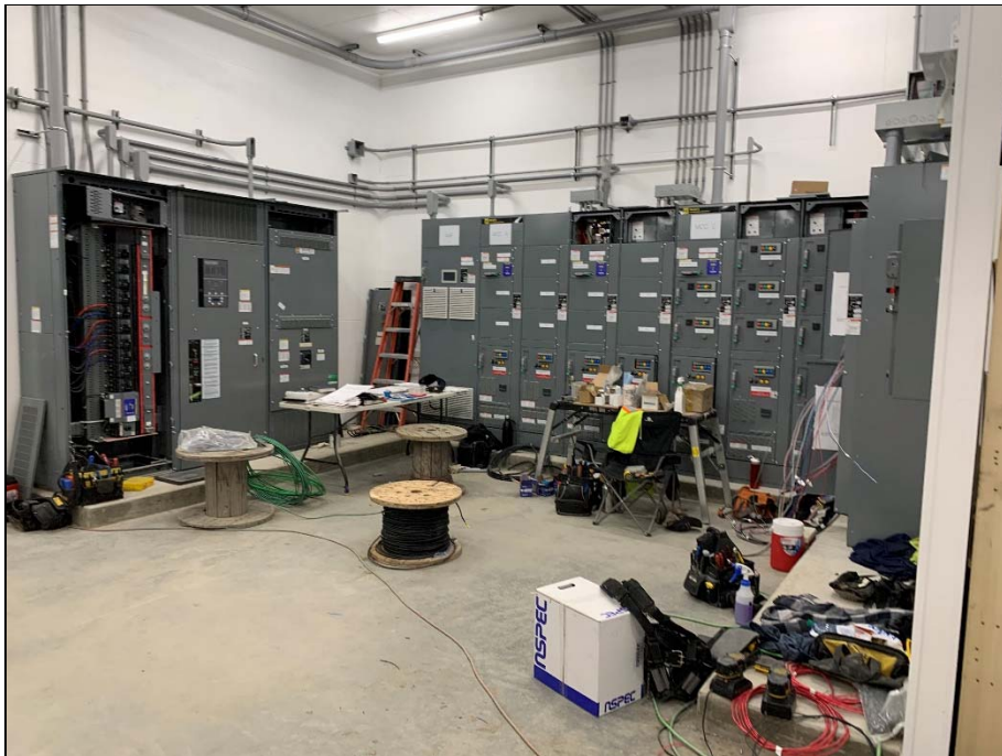
Significant progress on wiring to MCC.
