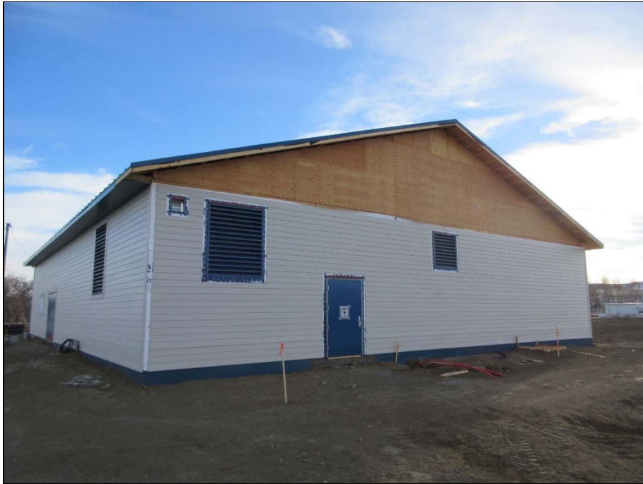
West side of water treatment has remaining siding.
