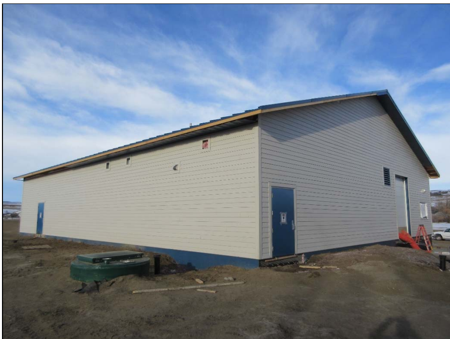
Rear of water treatment plant – siding and doors completed.
