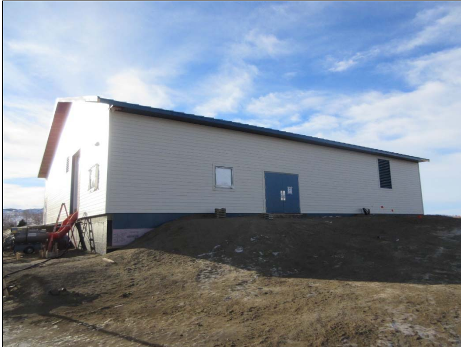
Front of water treatment plant – siding and doors completed.
