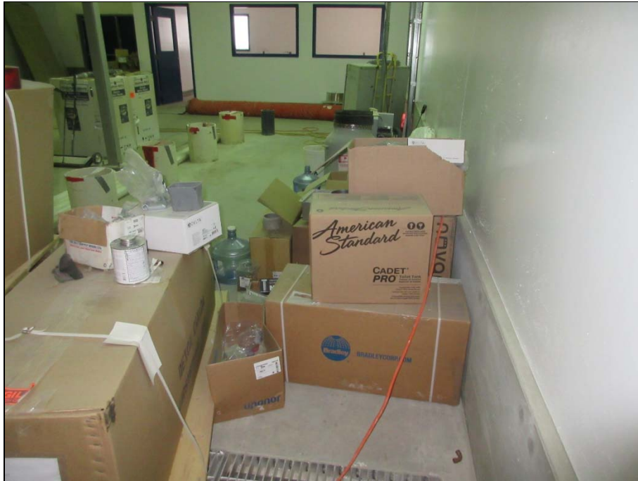
Additional mechanical material on site.
