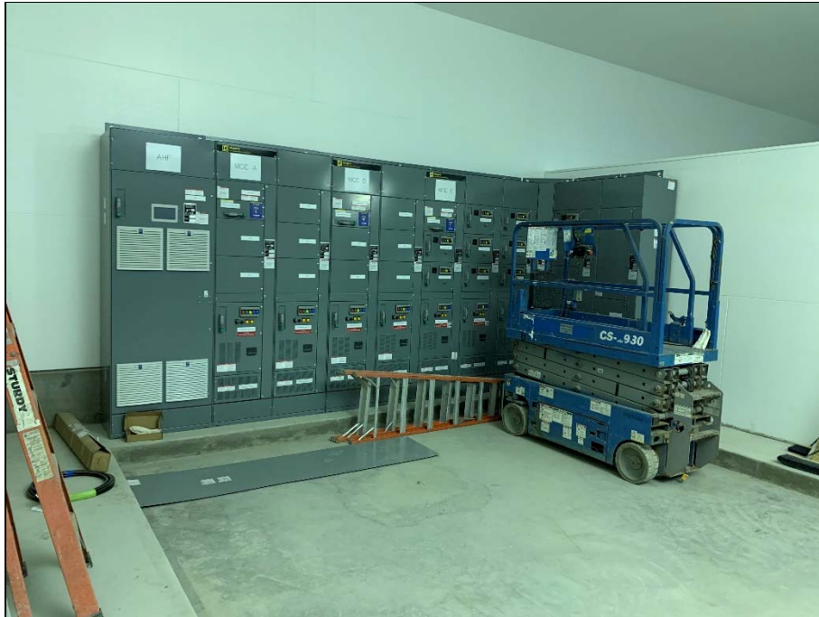
Motor control centre sections in place.
