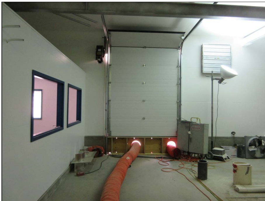
Overhead door and temporary heating ducts.
